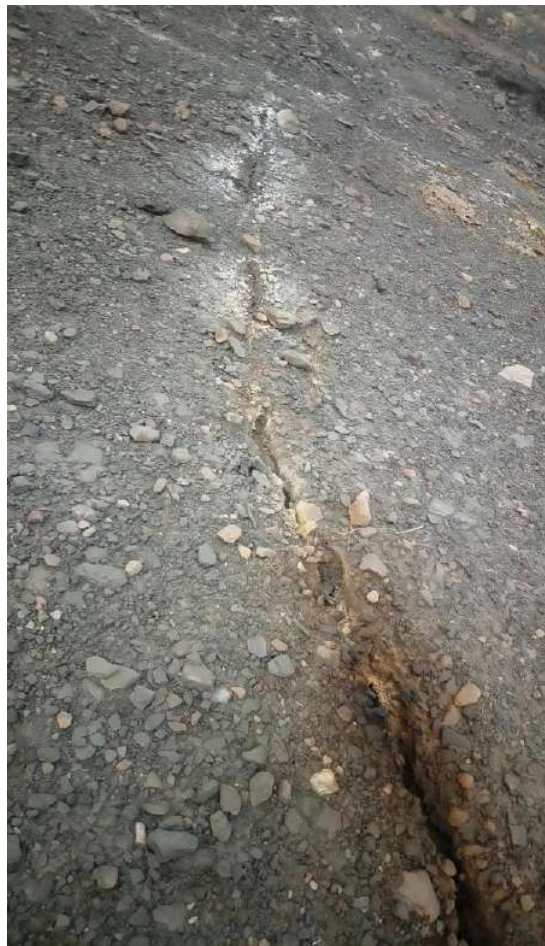
Figure 20: Fume cracks in the Bhulanbarari area.
