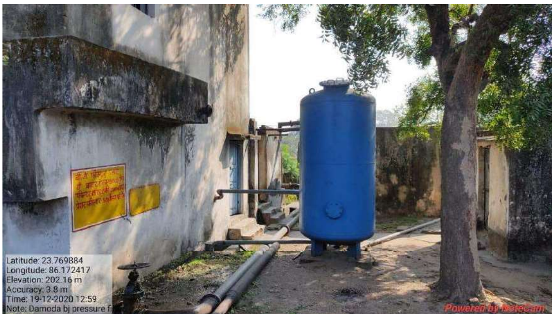
FILTER PLANT IN THE MINE AREA
